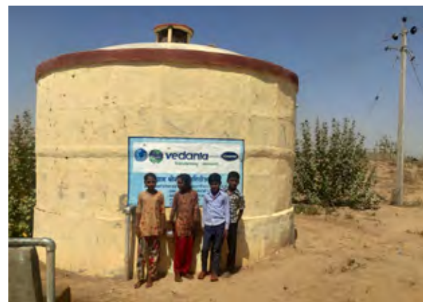
Community members at borewell constructed by Cairn
